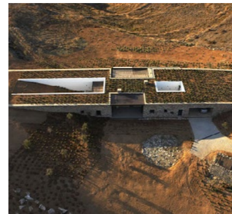
Example of earth sheltered structure
