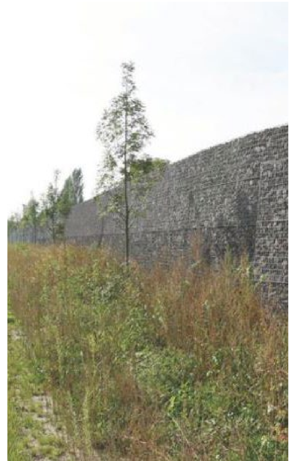
Using planting to integrate a gabion structure into the landscape
