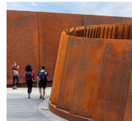
Example of weathering steel
