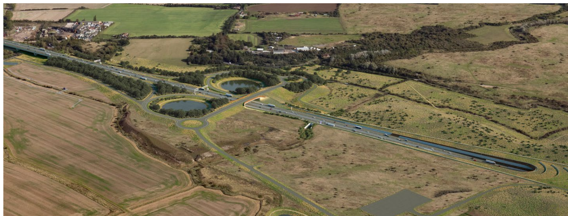
Illustrative views of the North Portal operational access bridge
