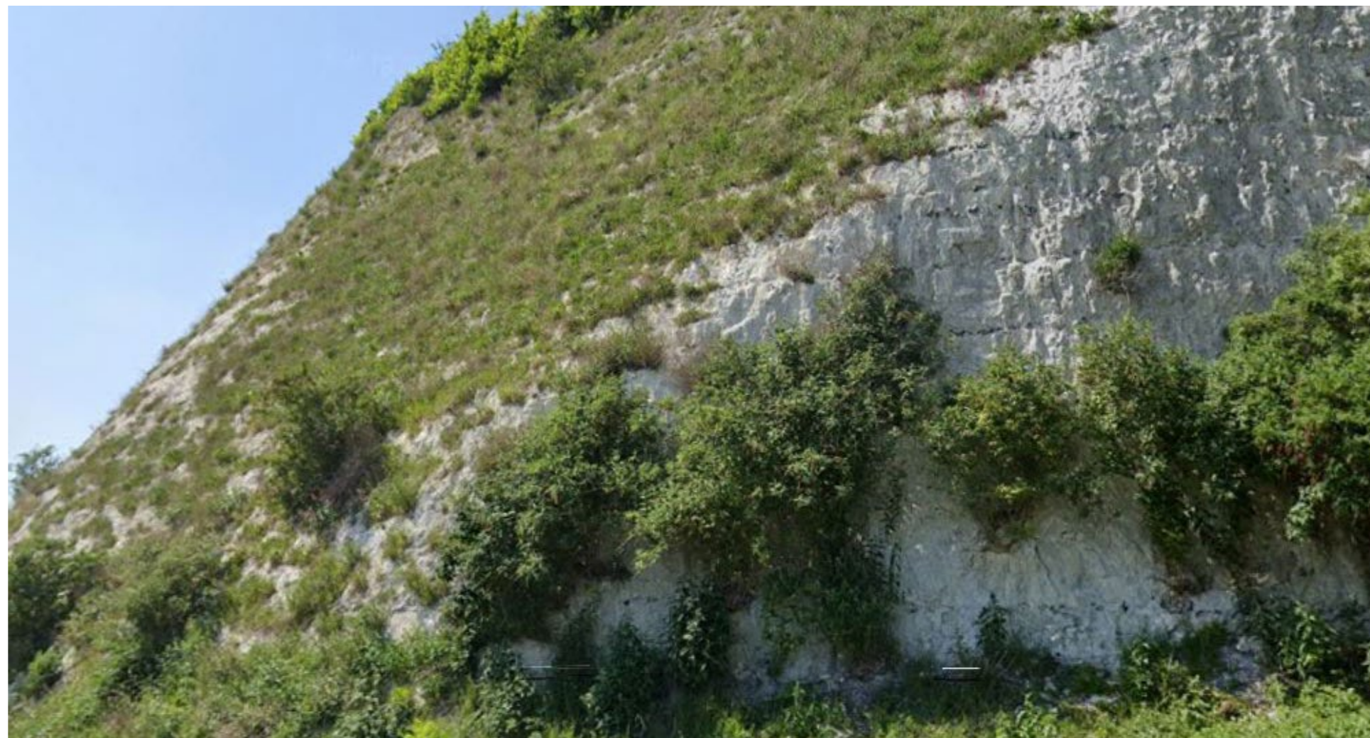
Example of a steep chalk cut with an irregular cut face
