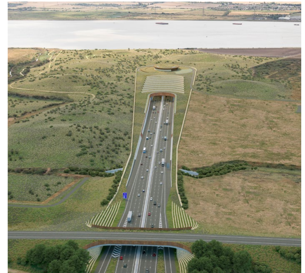
Illustrative view of the North Portal and North Portal operational access bridge
