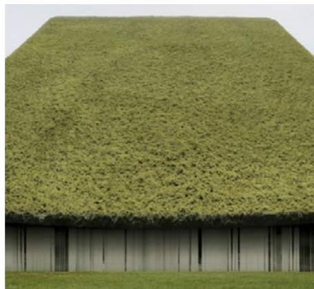
Example of green roof
