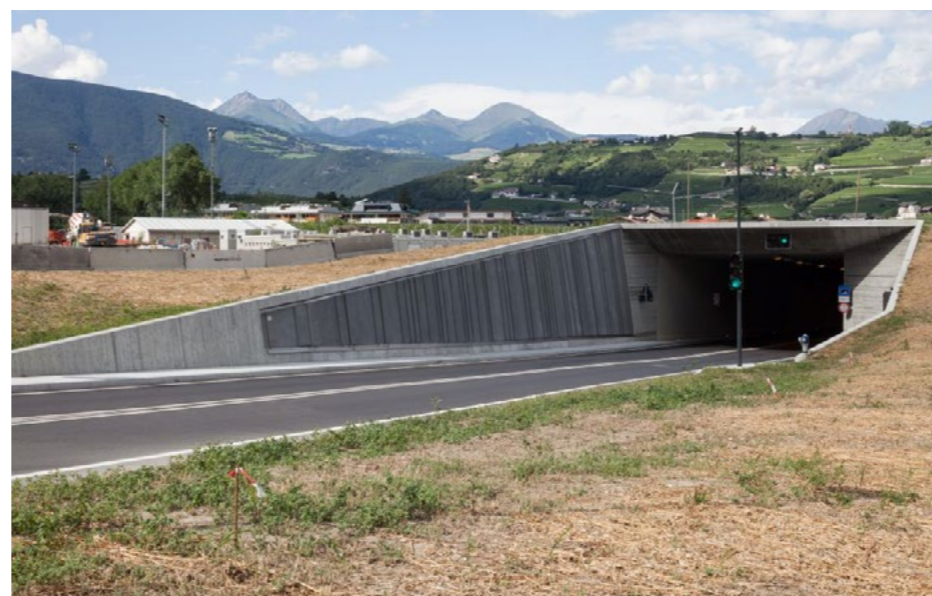
In situ concrete
