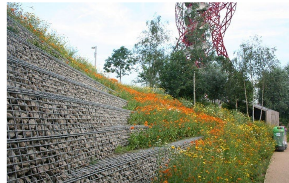
Gabions filled with local stone
