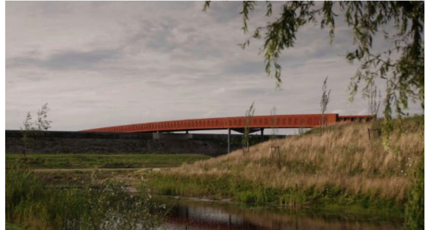
Example of using the structure to form the parapet and integrate graphics
