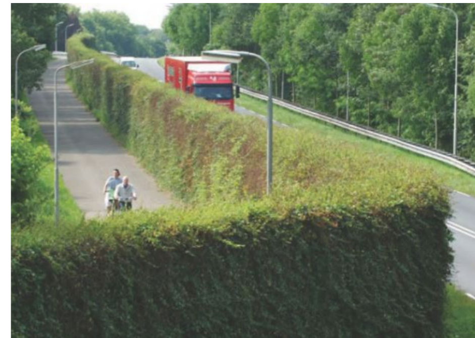
A green wall structure which separates a public access route from the highway
