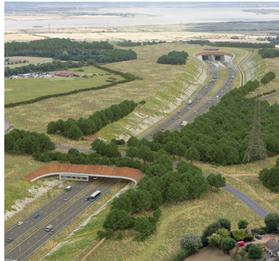
Illustrative view of the South Portal and Thong Lane green bridge north
