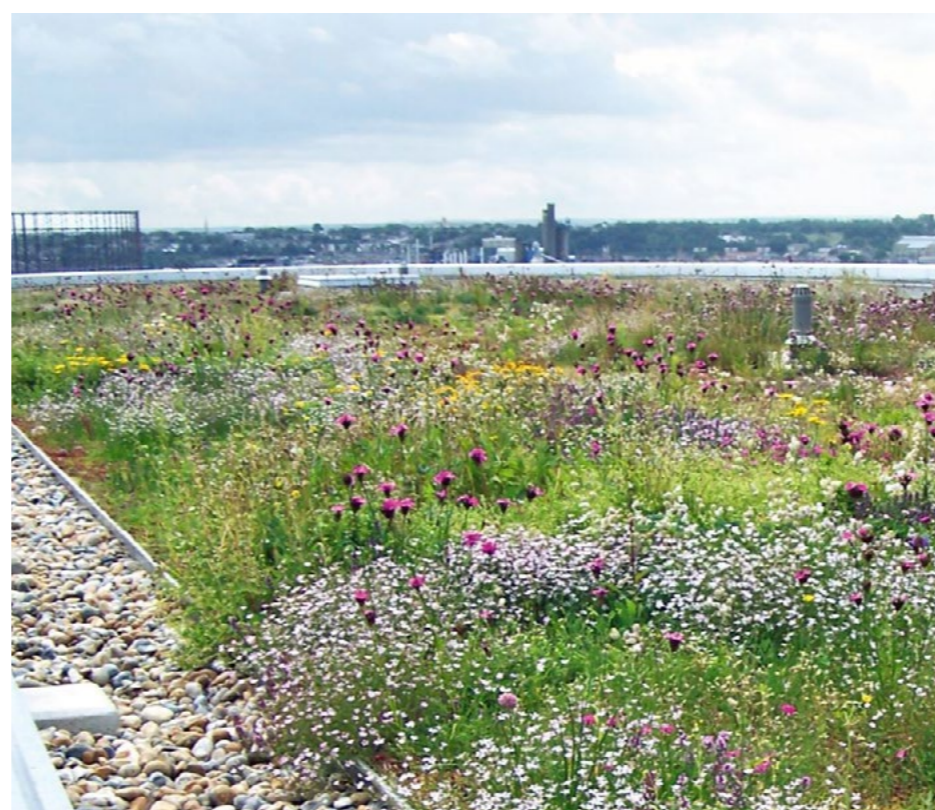
Example of an extensive green roof with planting
